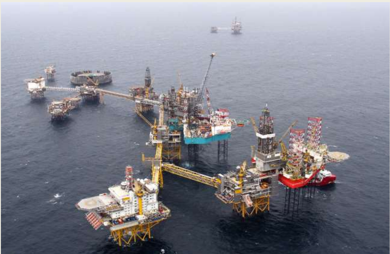
The Ekofisk platform. The nearest platform (with the helipad) is also the accommodation platform and includes an examination room. Photo: ConocoPhillips
