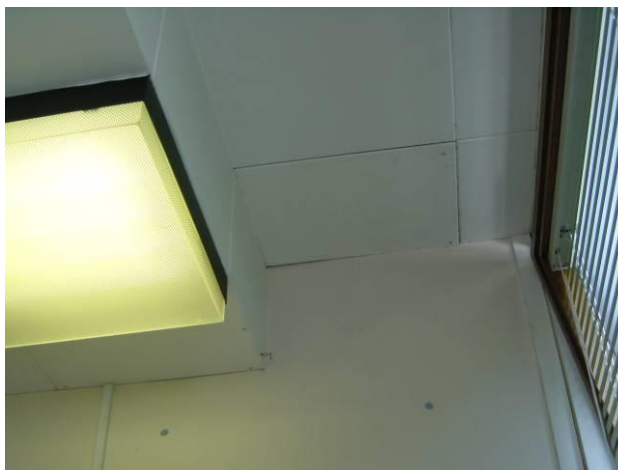
Figure 8.3 Asbestos insulating board ceiling tiles
