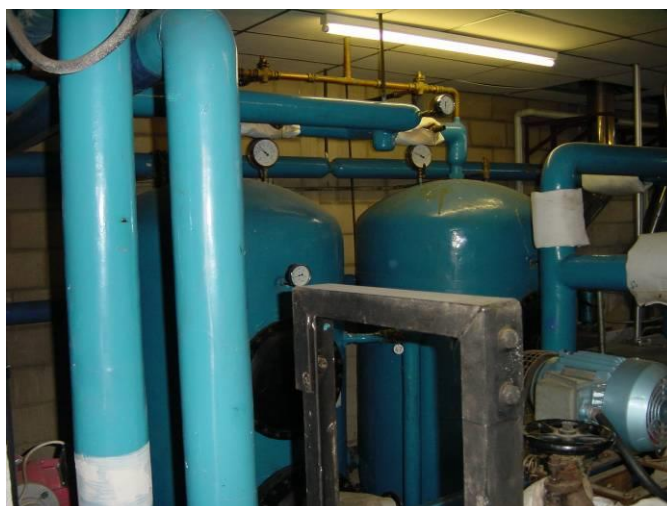
Figure 8.2 Insulation (lagging) to pipework and calorifiers
